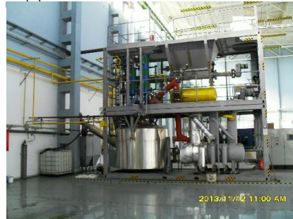
Switched operation solution, did not appear on the
